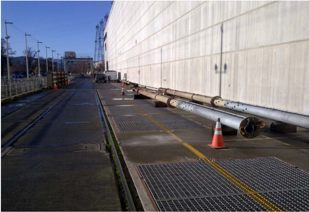
Collection channel pumps on tailrace deck for rehab.
